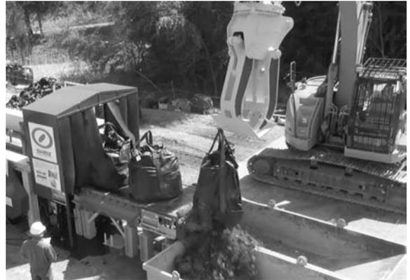
Fig. 5 Removing soil by a grapple attachment
